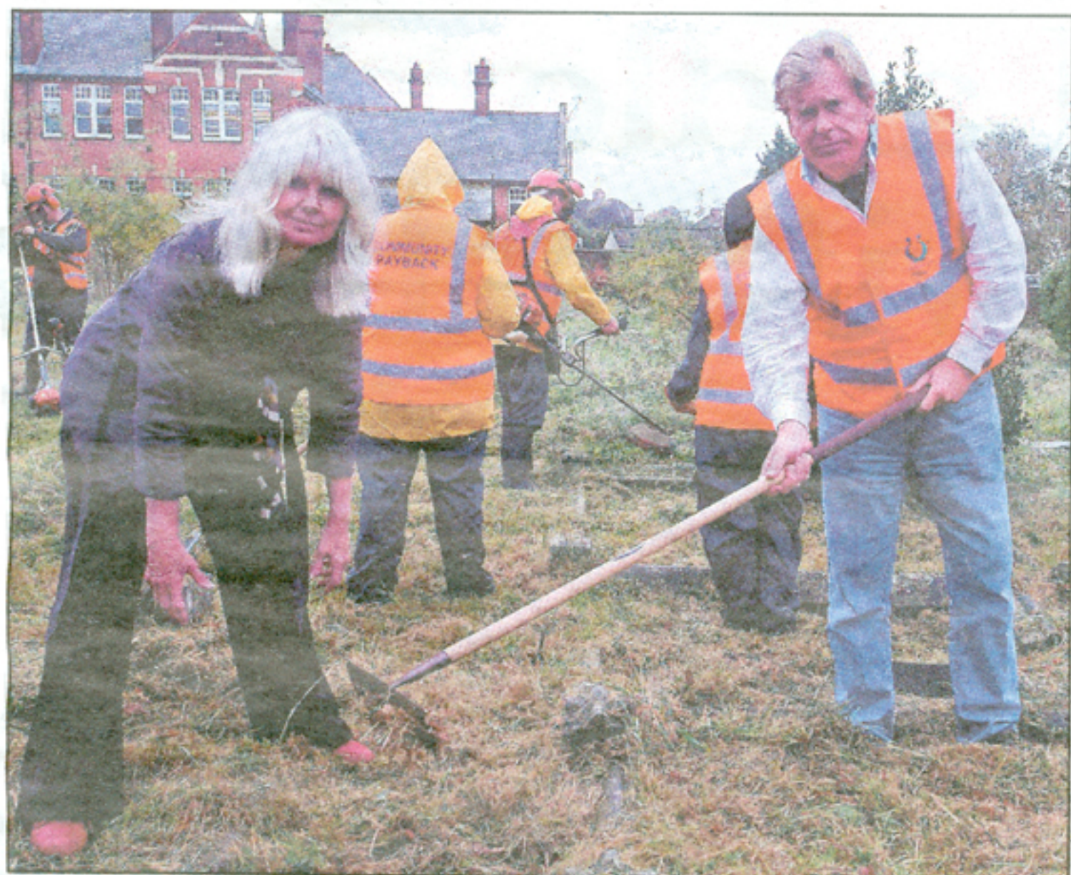
HARD AT WORK: Simon Burns MP, right, with Essex Probations Communication Officer, Lynn McKay and ex-offenders as they clear up the churchyard at Holy Trinity Church, Springfield
